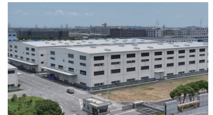
AST Production Plant (Centrifugal Compressor)
